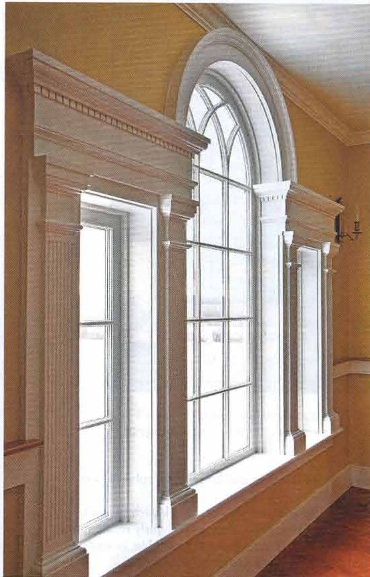
Connor Homes designed this Palladian window for a home in New York using classical detailing such as dentil molding and fluted pilasters.
