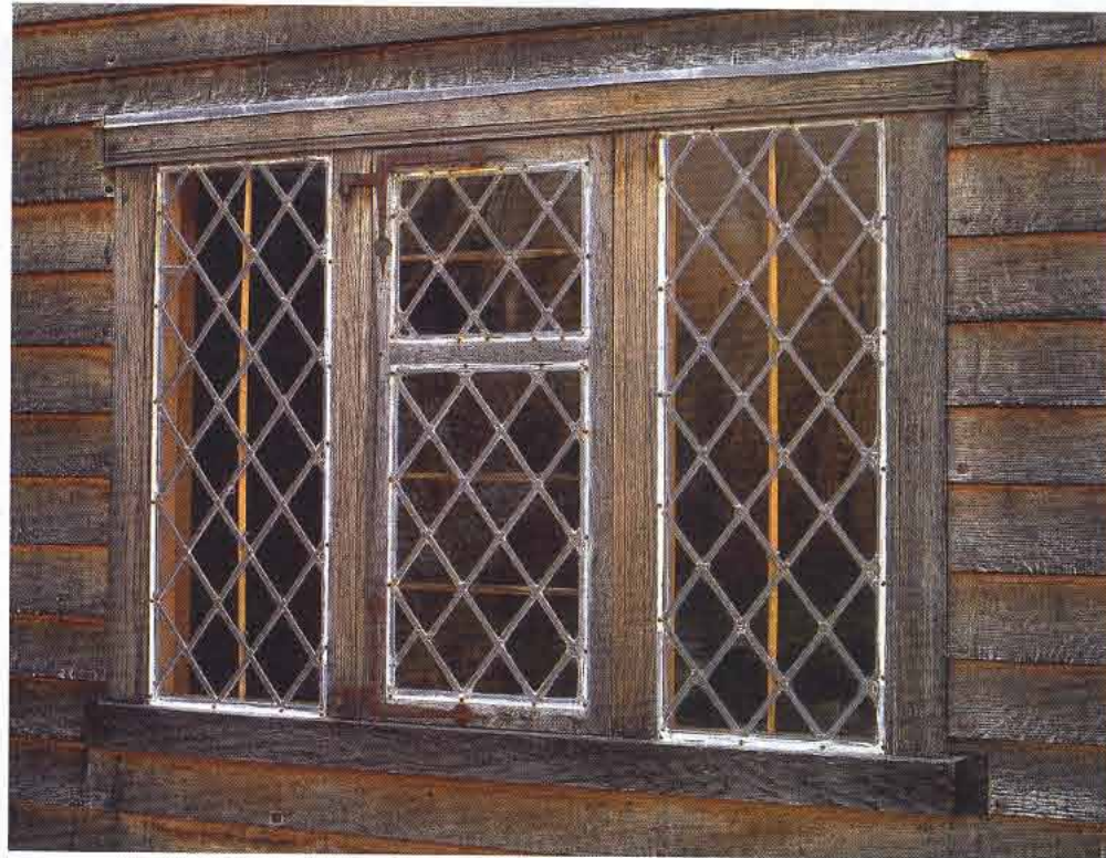
Maurer and Shepherd Joiners makes historically accurate windows, such as this seventeenth-century lattice window with diamond panes.
